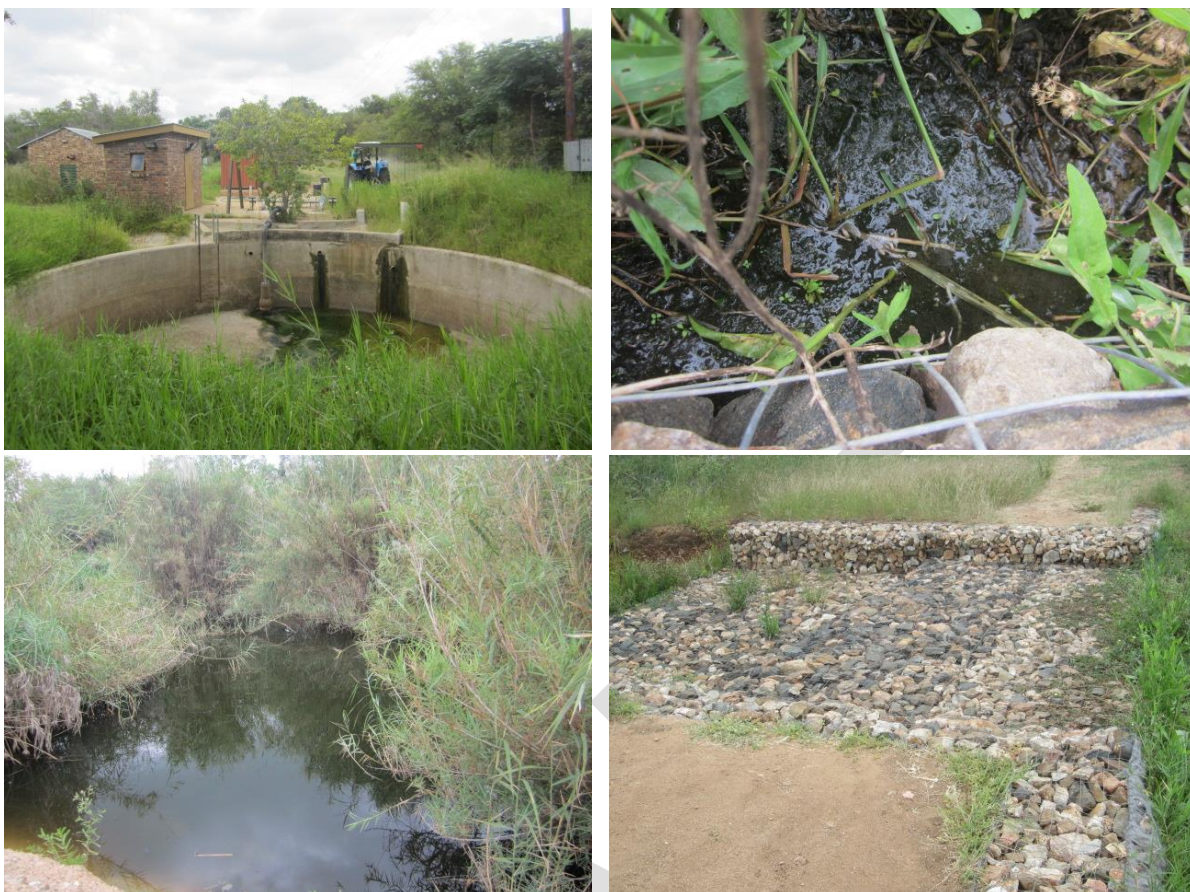
Plate 1: Photographs of water drainage and attenuation structures on site
