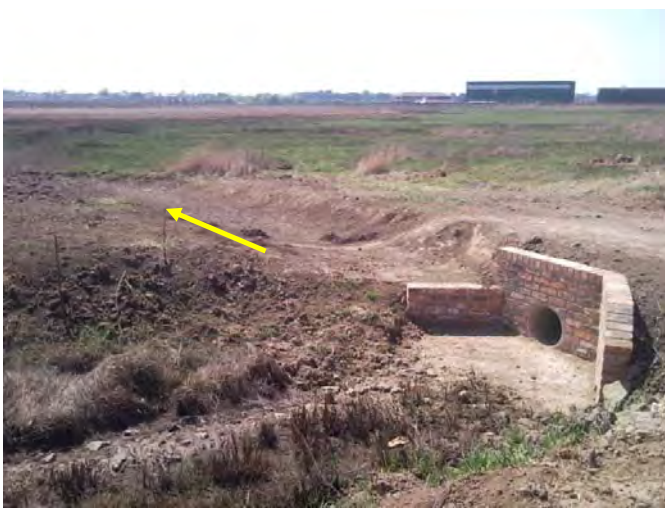
Overflow design with low spillway to direct the high rainfall events into the pan to minimize downstream impacts
