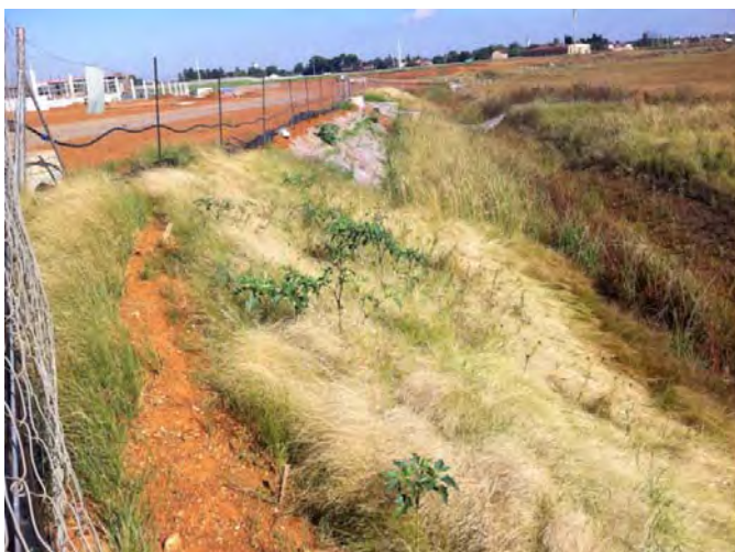
First hydro-seeding undertaken in 2010
