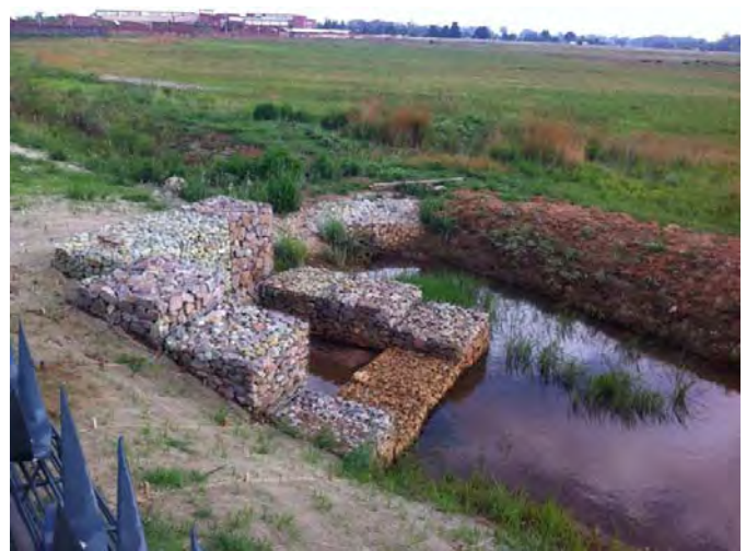
Gabion storm water structure with dissipation barrier from the commercial site (2011) .
