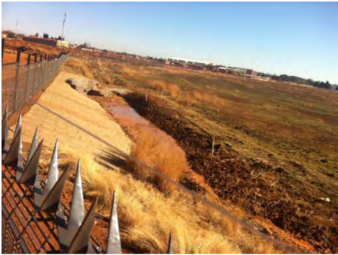
Rehabilitation of an embankment in the bio-swale using erosion control and hydro-seeding (2011)
